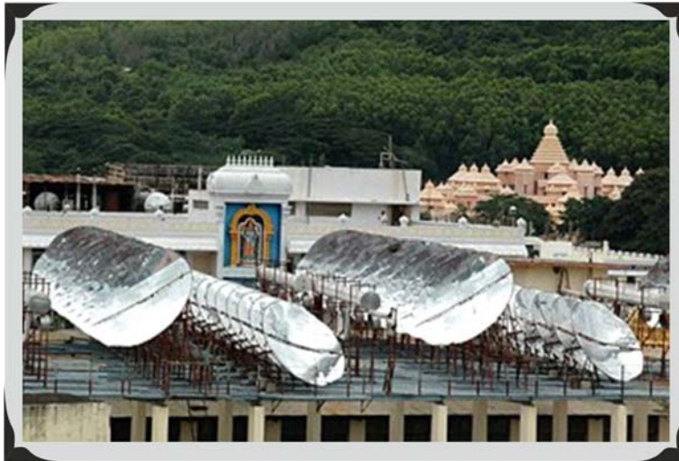
Figure 20 | Solar cookers atop the roof of the Lord Vishnu Temple, Tirumala, India.
